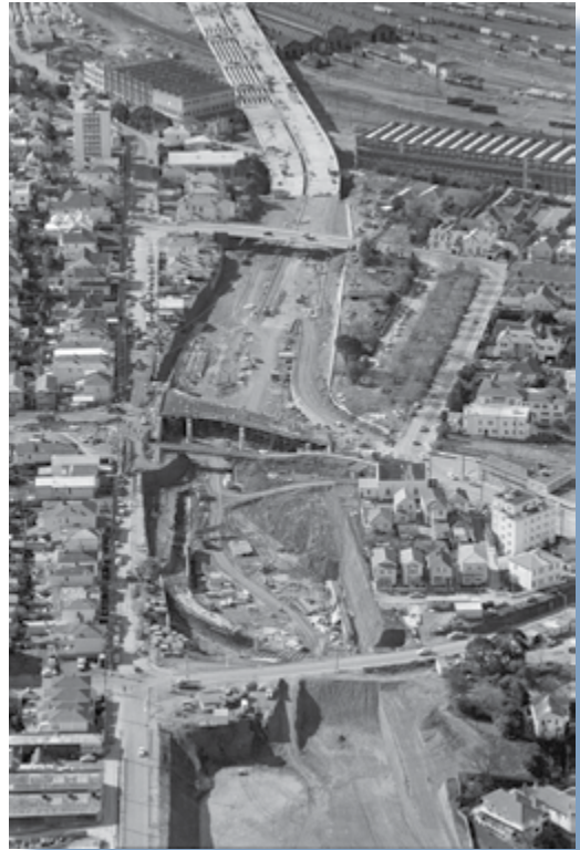
Photographer unidentified, ATL, Dominion Post Collection, EP/1969/3580/33.
